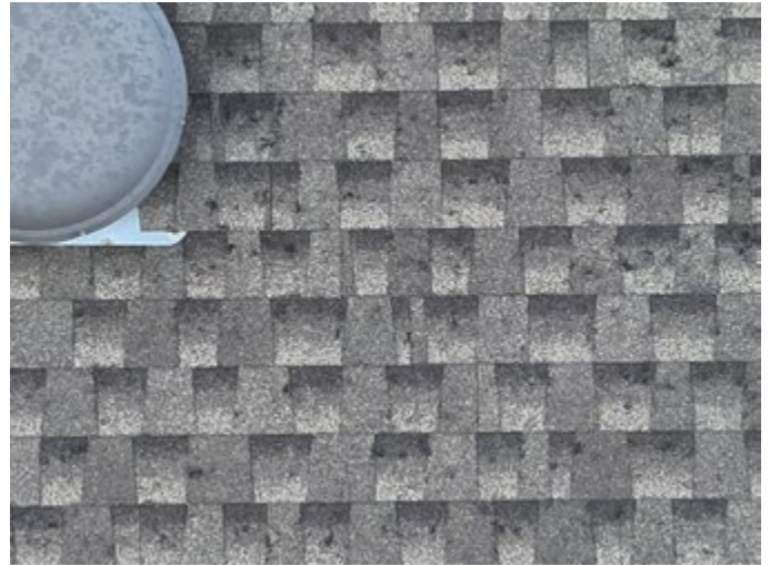
Non-Polymer Modified Asphalt Roof
