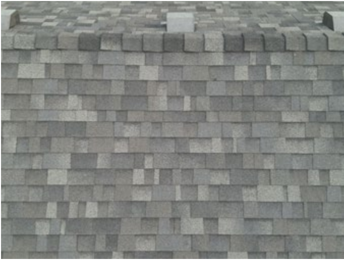
Polymer Modified Asphalt Roof
