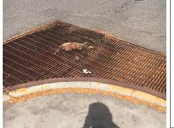
**2017-10: Storm Water Grate** The grate on the street corner outside the police department is being run over by vehicles and has become concaved. The edge of the grate is sticking up and is a potential trip and <u>fall</u> hazard. Replace the grate with one that is robust enough to handle vehicle traffic. Check all other similar storm water grates for damage and replace as needed.
